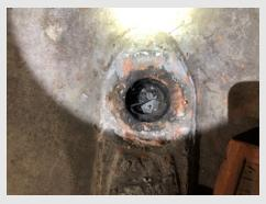
2) Note: There is a clean out that appears to be associated with the sewer line. This may be indicative of recent repairs made on the system.
