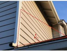
2) Hardiplank siding issue on south side. Installation concerns with the siding planks: 1) Nails have been used to secure the bottom edge and corners of the planks. This is not the proper installation and expansion of these boards will likely result in cracks and broken pieces of the siding. 2) Caulking has been used where joints are to be flashed and not caulked. Consult siding contractor for further evaluation, recommendations and repairs where needed.
