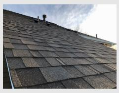
2.12 Type of material Composition laminated (architectural) shingle. This is usually considered a 25-30 year roofing material. Consult installer or manufacturer for further information on roofing warranty.
