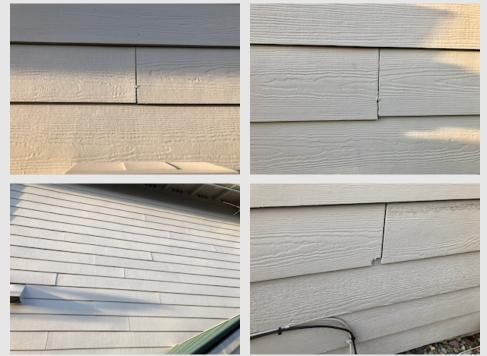
Some maintenance caulking recommended with the siding there are fastener holes and penetrations in the siding. Seal all penetrations in siding to protect from moisture. Wood trim. No issues observed.
