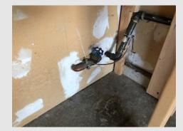
\* Closing this valve will shut off the water supply to the whole house. It is recommended that this be labeled and kept easily accessible.
