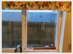
2) Vents are present in the window frame. These provide a valuable source of fresh air into the house in conjunction with the ventilation fan system. It is recommended that these vents remain open to ensure a regular air exchange within the house.
