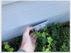
2) Missing receptacle cover screw in garage. This is a safety concern. Ensure all outlet receptacles have a properly secured cover in place.
